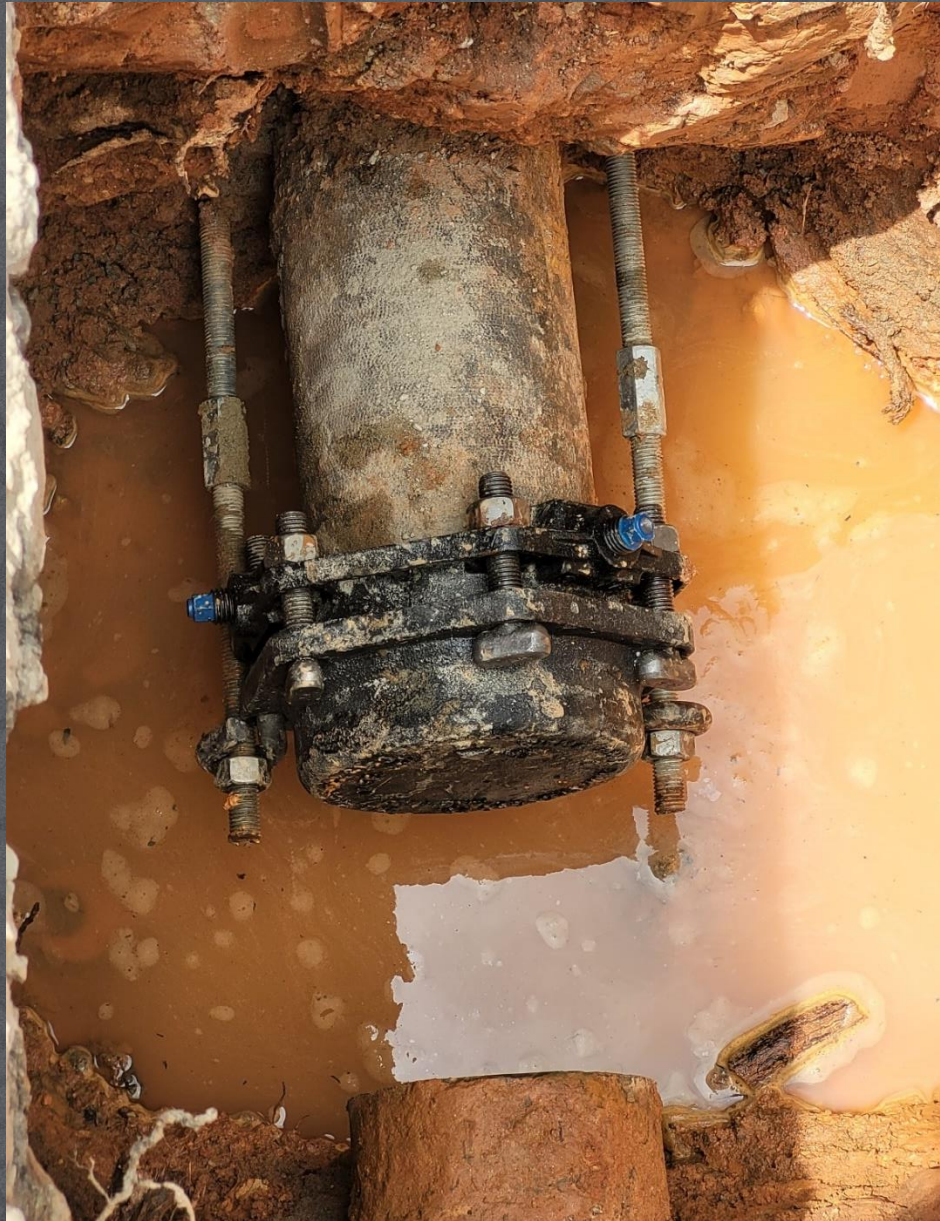
New Gordon Avenue Water Main Termination
