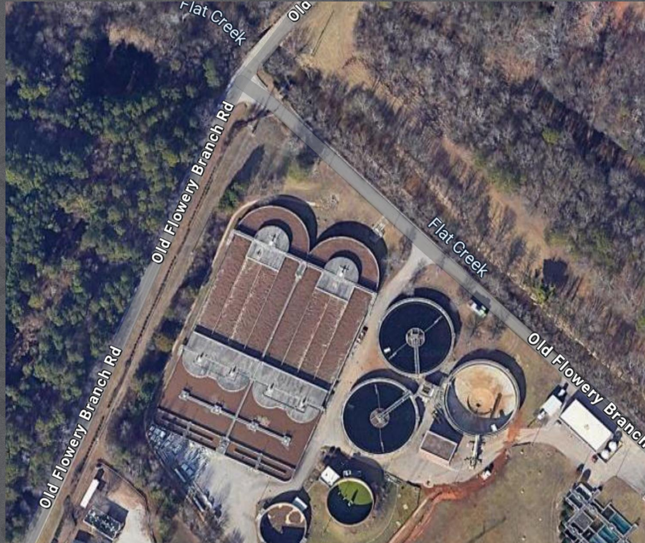
Flat Creek WRF Aeration Basins and Clarifiers
