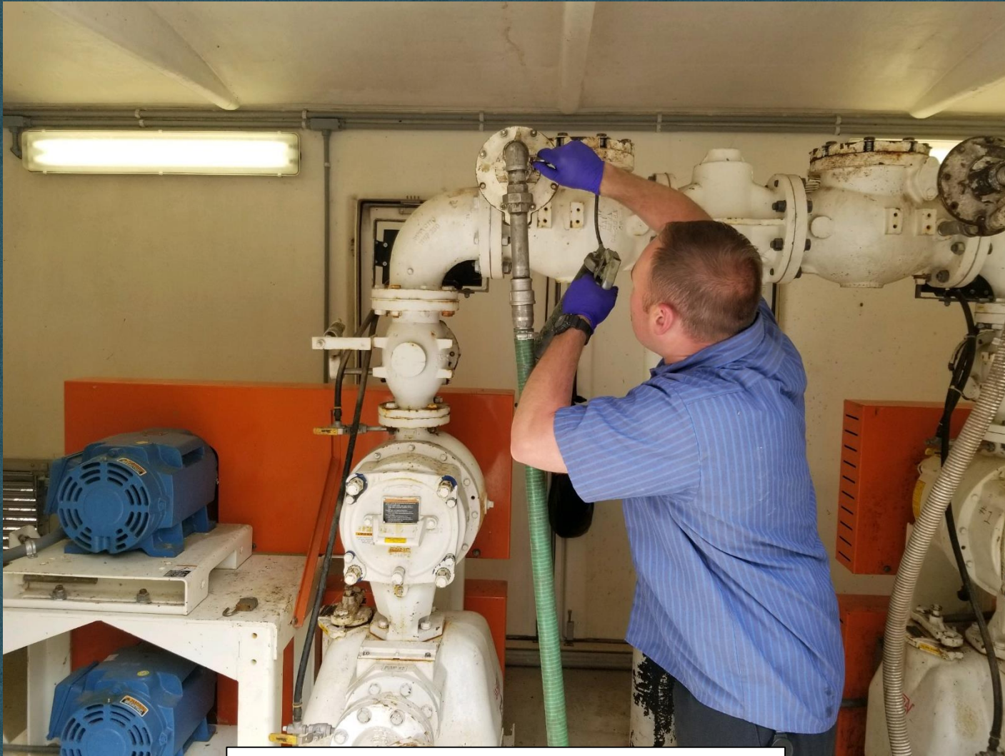
Lift Station Maintenance
