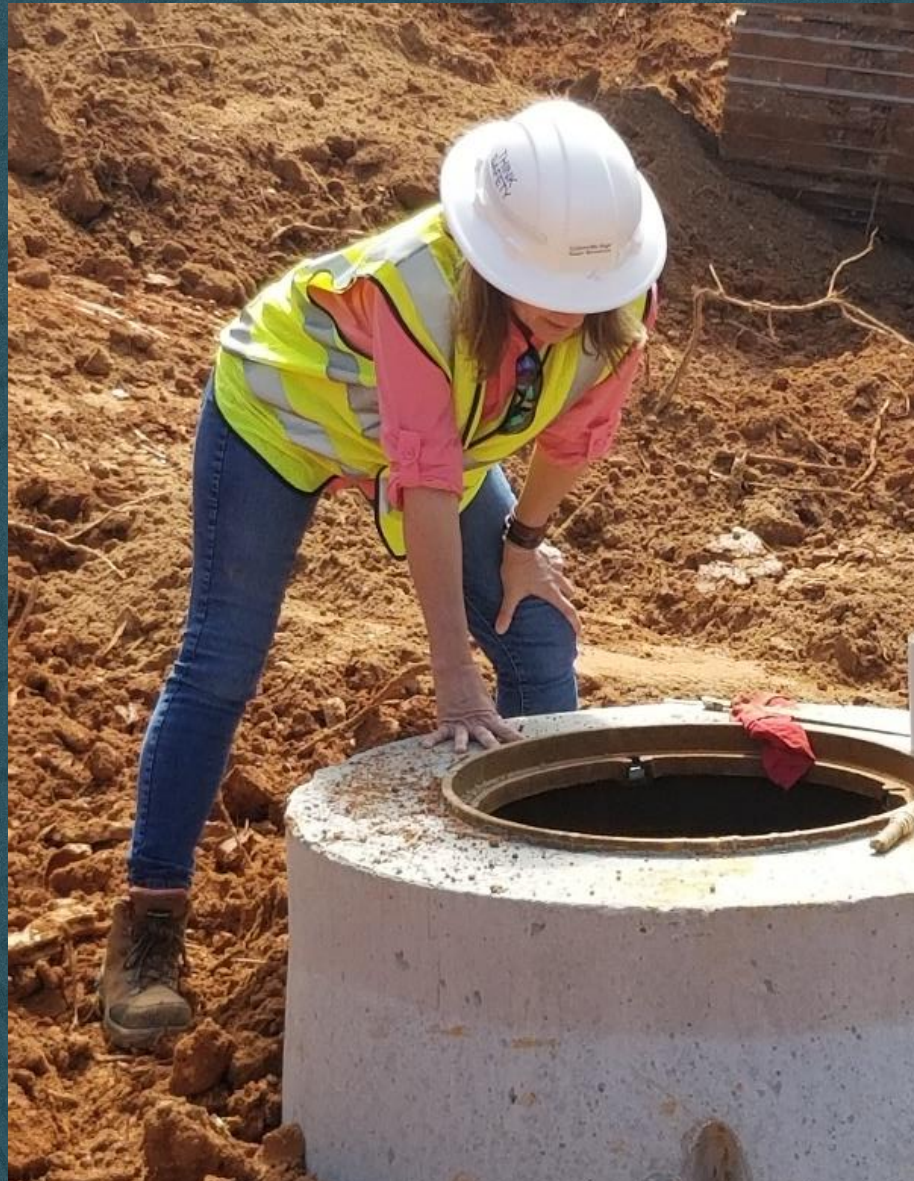
Gravity Sewer Manhole Construction on Webb Girth Road
