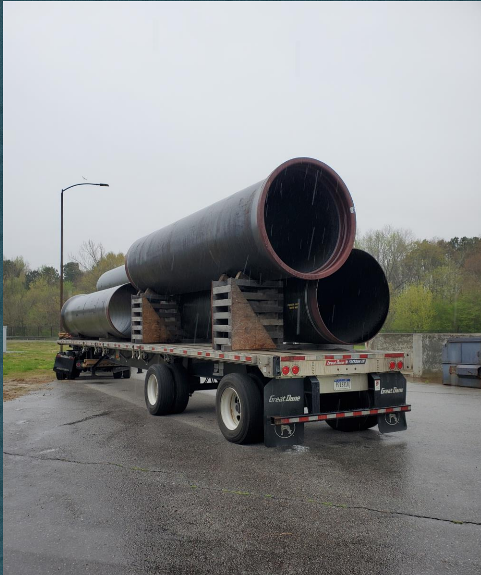
54- and 64-Inch Protecto 401 Lined Ductile Iron Sewer Pipe for Flat Creek WRF
