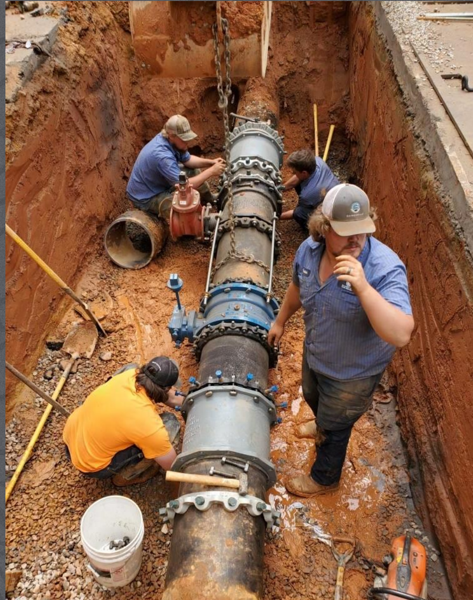
DWR Crews Repair a Large Diameter Water Main
