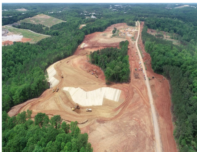
85 Business Park Construction
