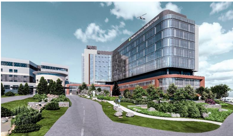
Northeast Georgia Health System is under construction on a new, multi-story patient tower, at the NGMC Gainesville campus. The new Patient Tower in Gainesville will be a 927,000-square-foot expansion that will make NGMC Gainesville the third-largest hospital in Georgia (by beds).
