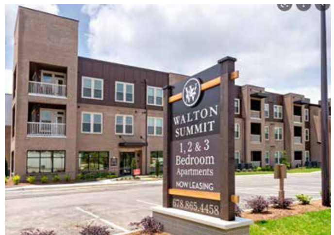
Example of a multi-family building
