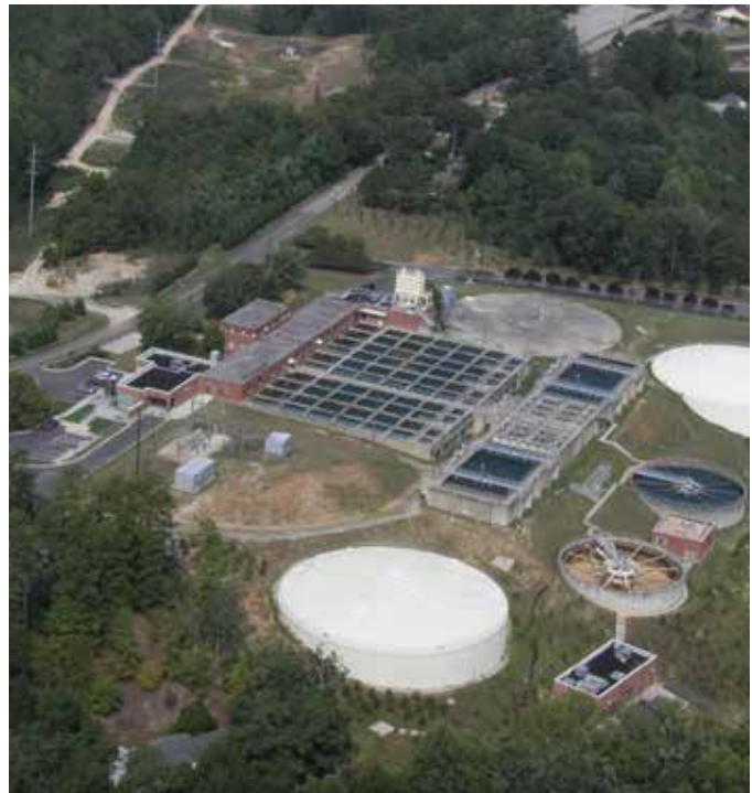
Riverside Water Treatment Plan
