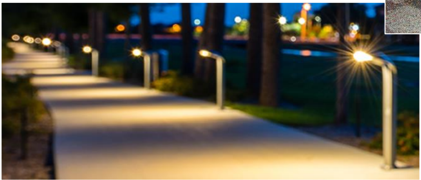
Rock Creek Greenway Lighting
