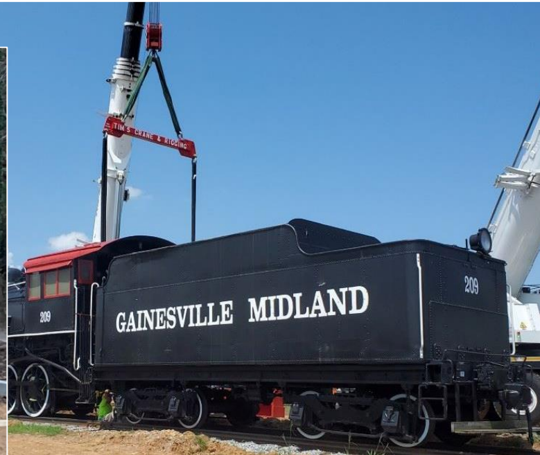
Engine 209 Park Relocation
