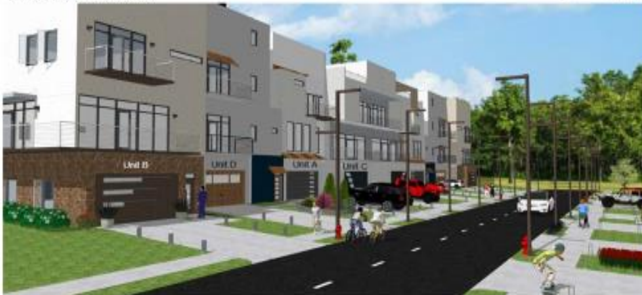
Looking at Limestone Parkway side.
