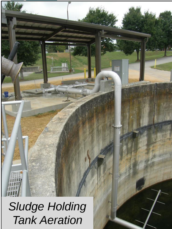
Sludge Holding Tank Aeration
