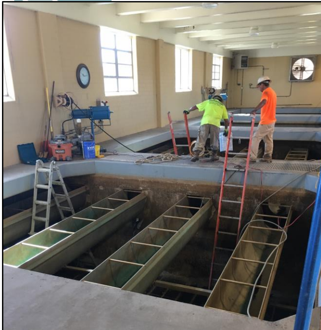
Riverside WTP Filter Media and Underdrain Replacement
