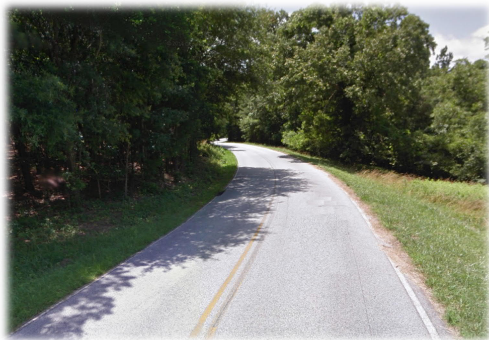
Photograph 17 – Lakeview Drive Along Site Frontage Facing South
