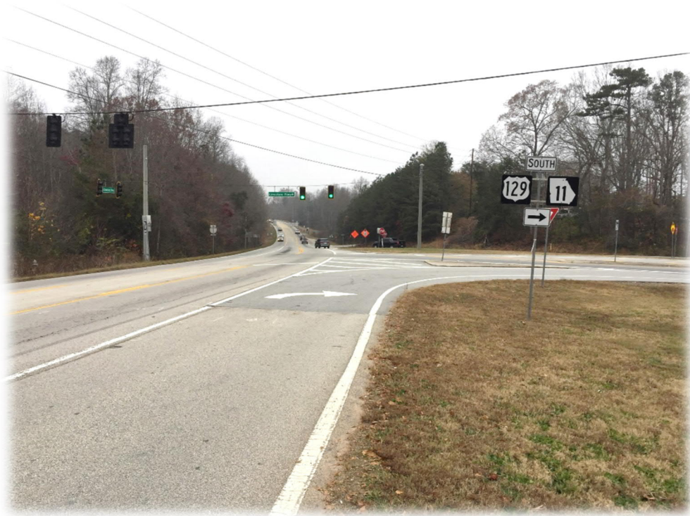
Photograph 1 – Cleveland Highway Facing North at Limestone Parkway
