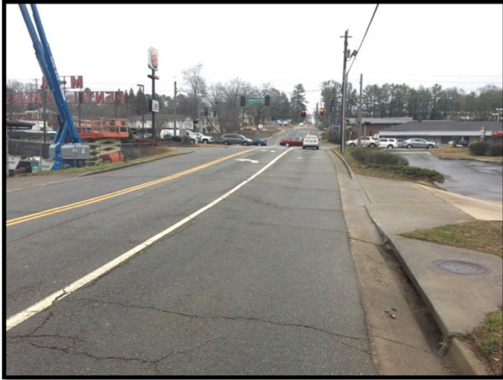
Photograph 4 – Enota Avenue Facing East Toward Thompson Bridge Road, Site Access to Right
