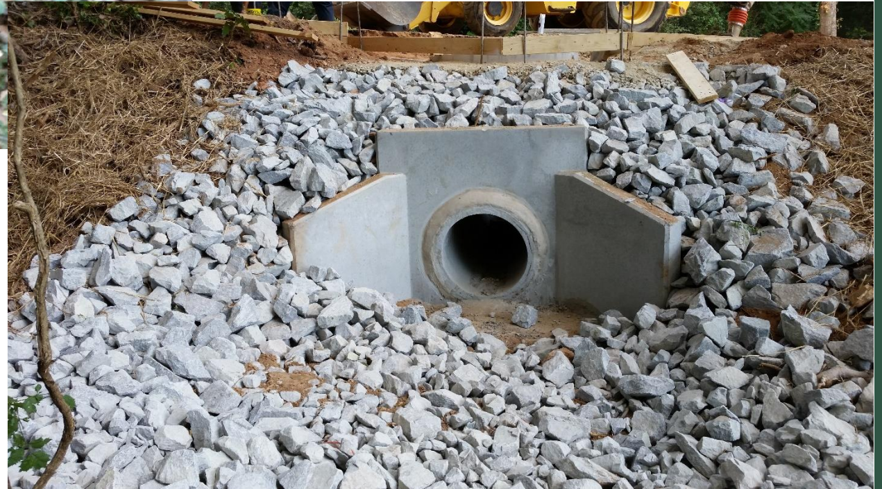
“After”: Head wall and stone installation.
