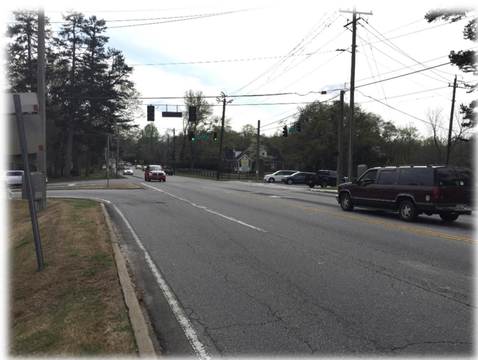
Photograph 15 – Park Hill Drive at South Enota Drive
