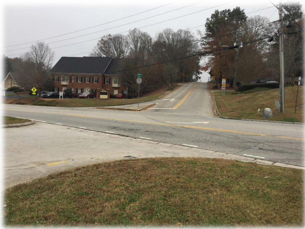
Photograph 14 – South Enota Drive Facing Robinhood Trail
