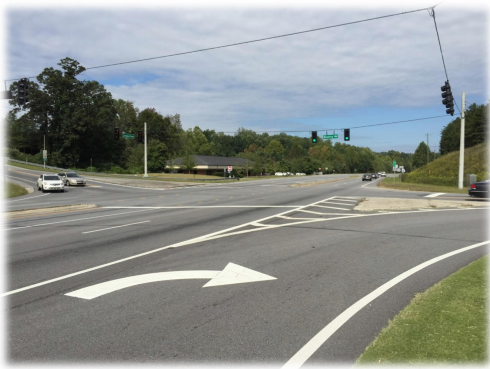
Photograph 3 – Limestone Parkway at Beverly Road Facing Northwest
