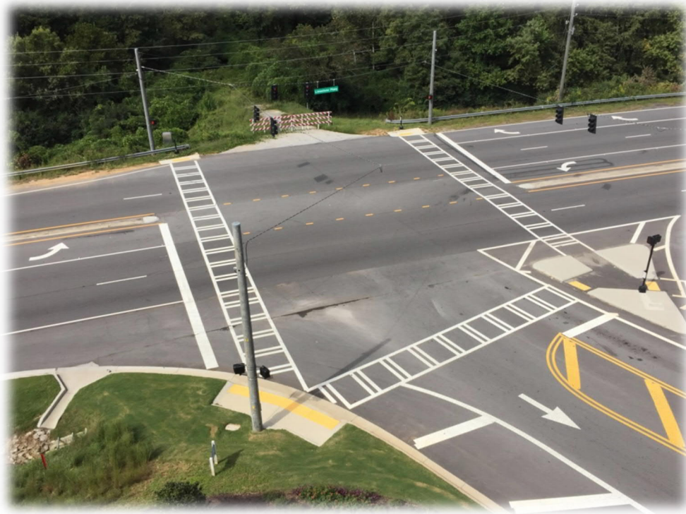
Photograph 4 – Limestone Parkway at Kroger Access Facing West Toward Subject Site
