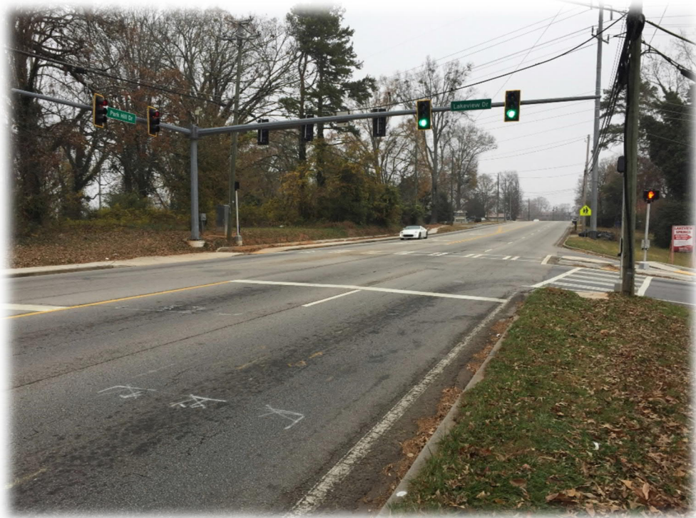
Photograph 16 – Park Hill Drive at Lakeview Drive
