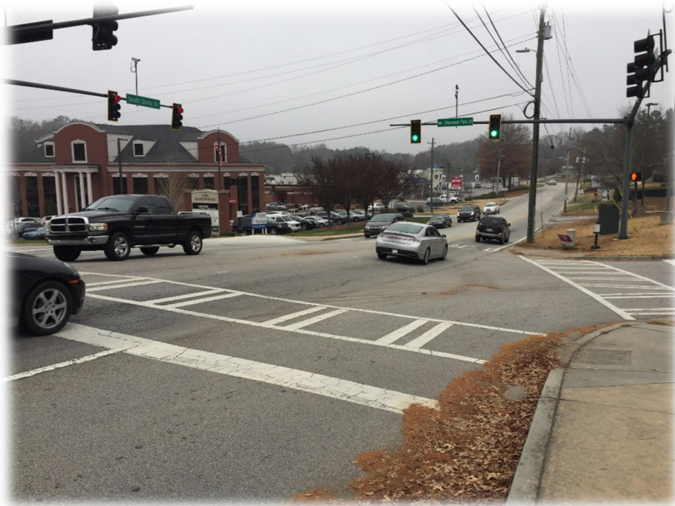
Photograph 13 – South Enota Drive Facing North at Sherwood Park Drive
