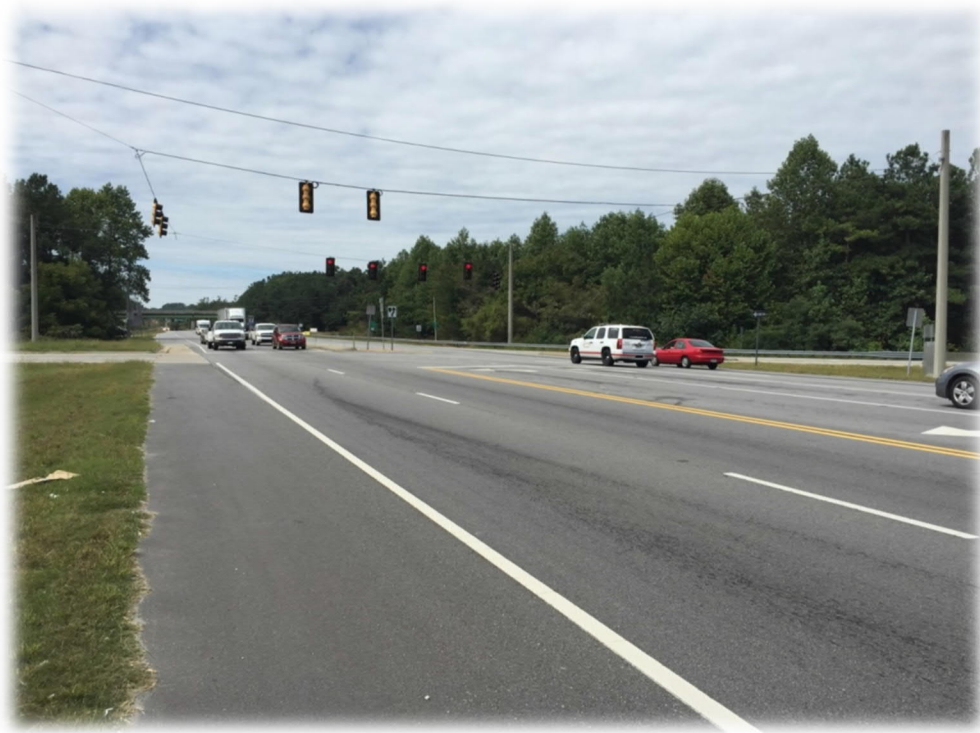
Photograph 7 – Jesse Jewell Parkway at I-985 Southbound Ramps Facing West
