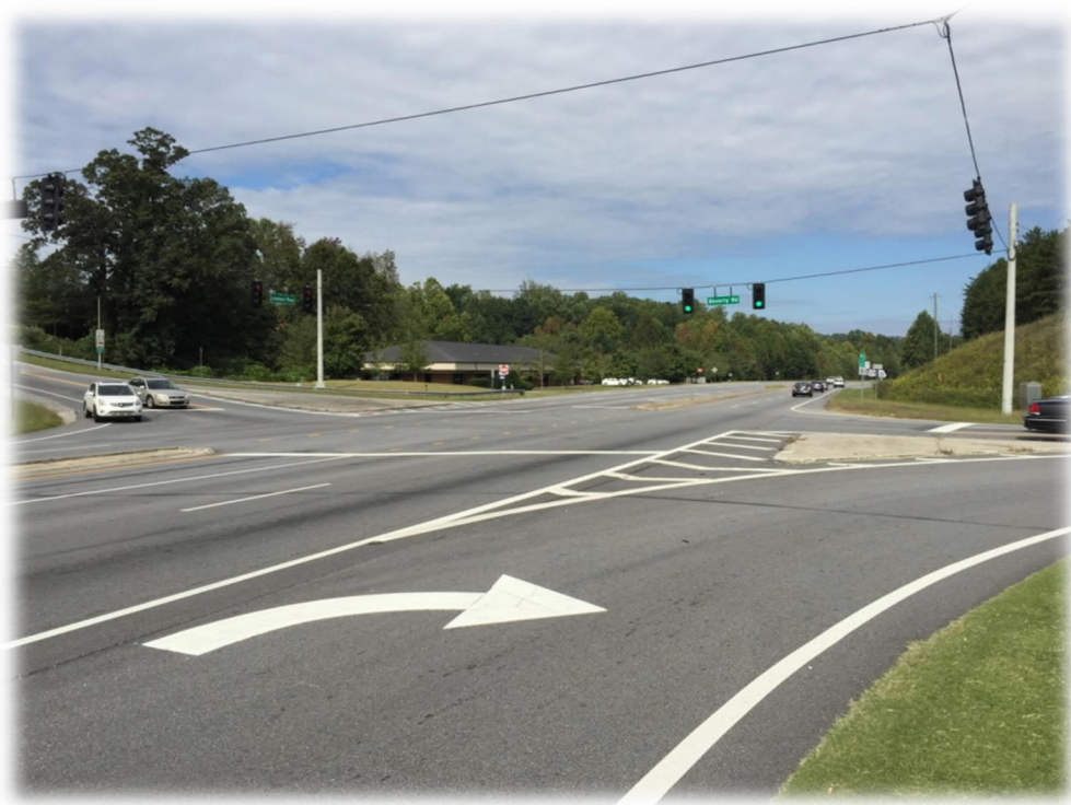
Photograph 3 – Limestone Parkway at Beverly Road Facing Northwest
