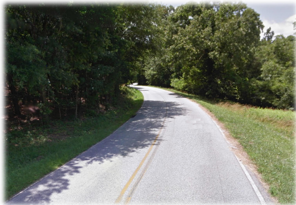
Photograph 17 – Lakeview Drive Along Site Frontage Facing South
