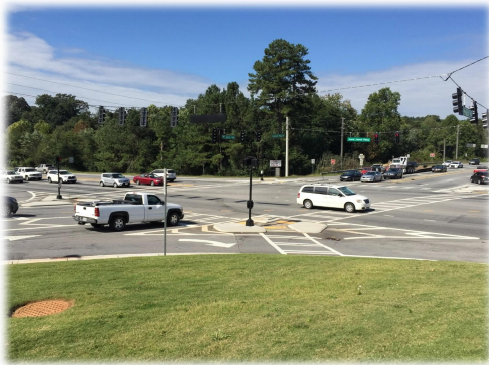
Photograph 5 – Limestone Parkway at Jesse Jewell Parkway Facing North
