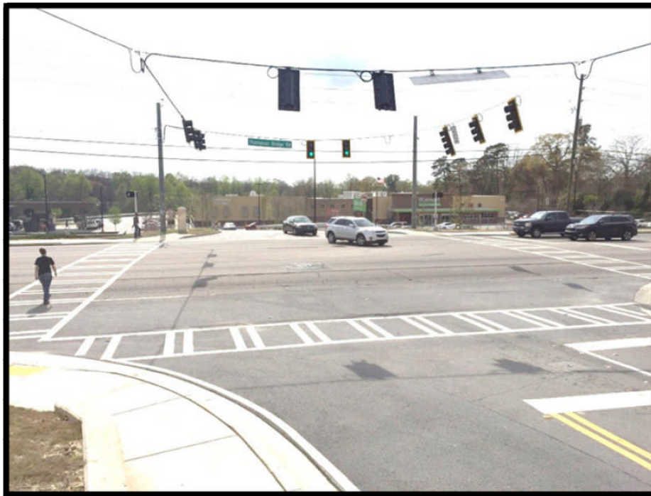
Photograph 1 – View of Thompson Bridge Road Facing Walmart from Taco Bell Access
