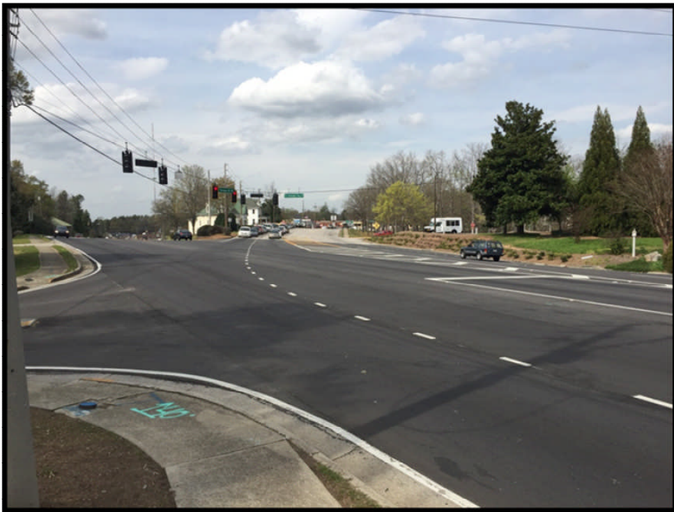
Photograph 7 – Green Street Facing North at Fork with Thompson Bridge Road to Left, GA 11 Bus to Right
