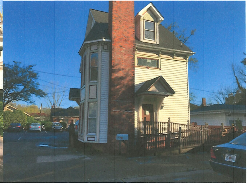
ATTACHED BUILDING: proposed for office space
