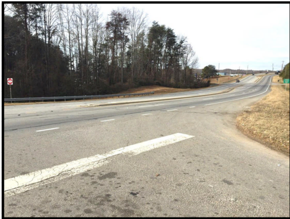
Photograph 2 – View From Sportsman Club Road Facing North Along GA 53
