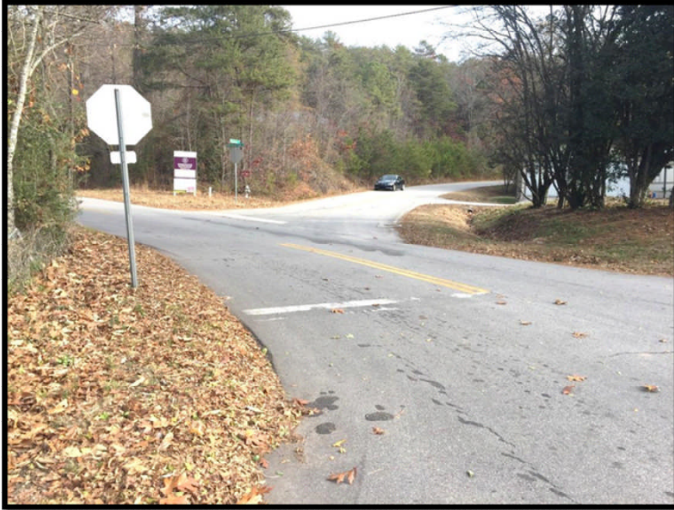
Photograph 1 – Sportsman Club Road Facing Strickland Drive From Old Dawsonville Highway
