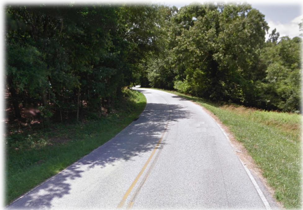
Photograph 17 – Lakeview Drive Along Site Frontage Facing South
