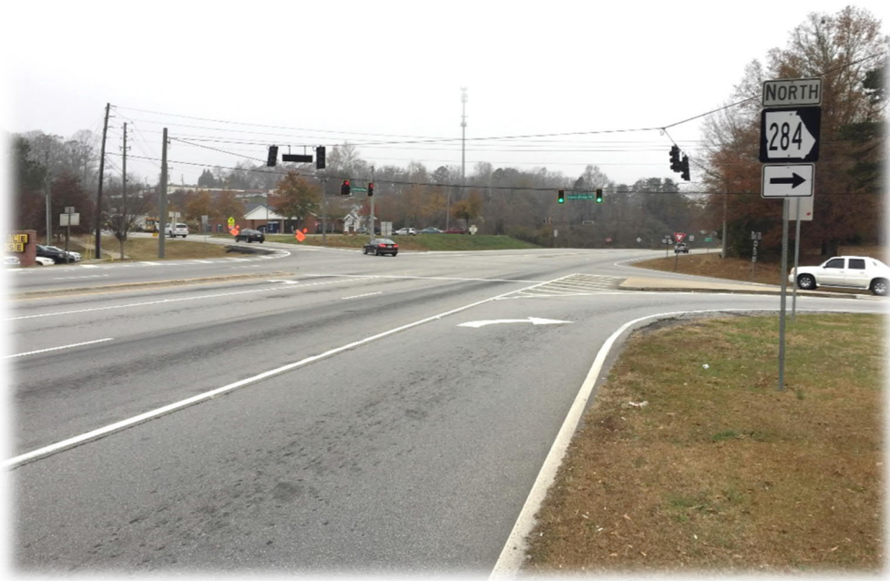
Photograph 2 – Limestone Parkway Facing North at Clarks Bridge Road
