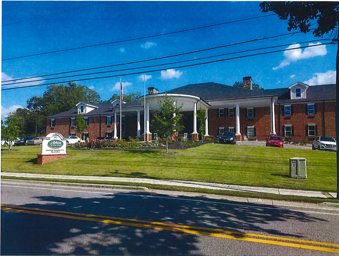
Existing Assisted Living Facility
