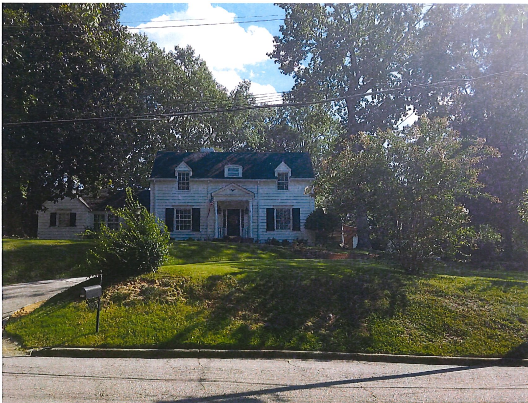
Existing Single Family Home
